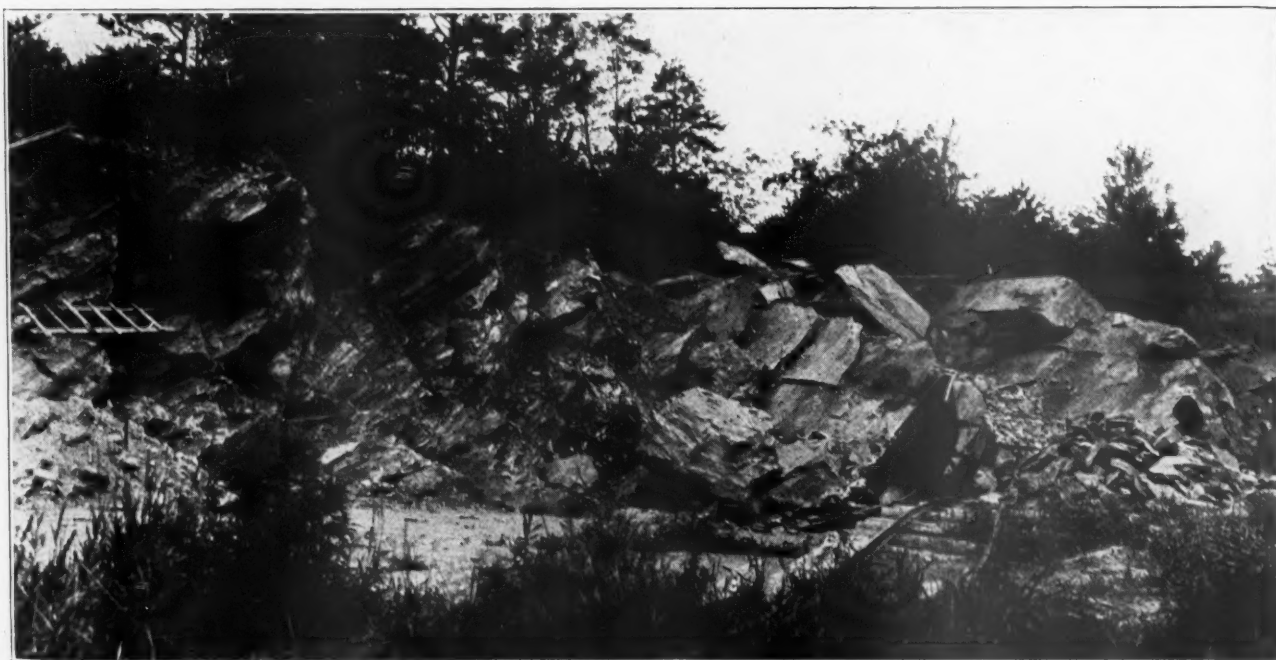
View of Quarry and Dump Car at Forgone and Romano
